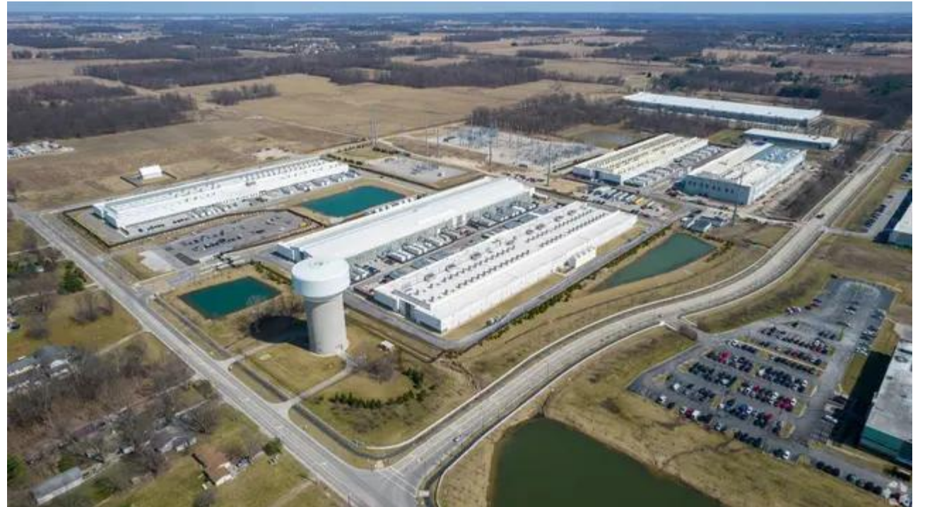
Amazon data center campus in New Albany, Ohio. (CoStar)
